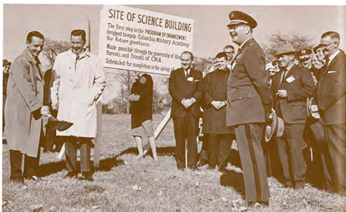
Construction site of Science Building
